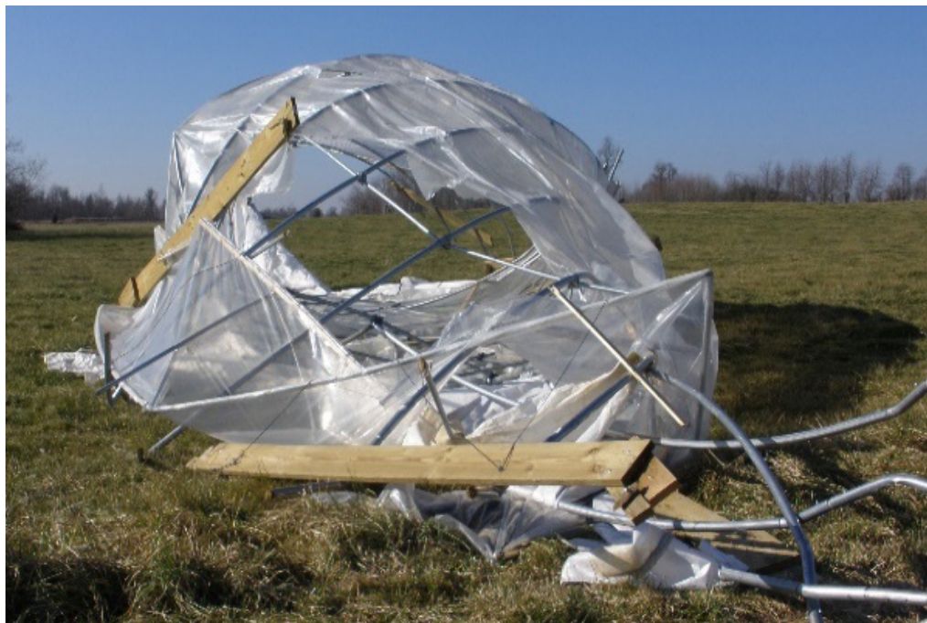
Figure 2. This high tunnel was destroyed after winds pulled it from the ground.
