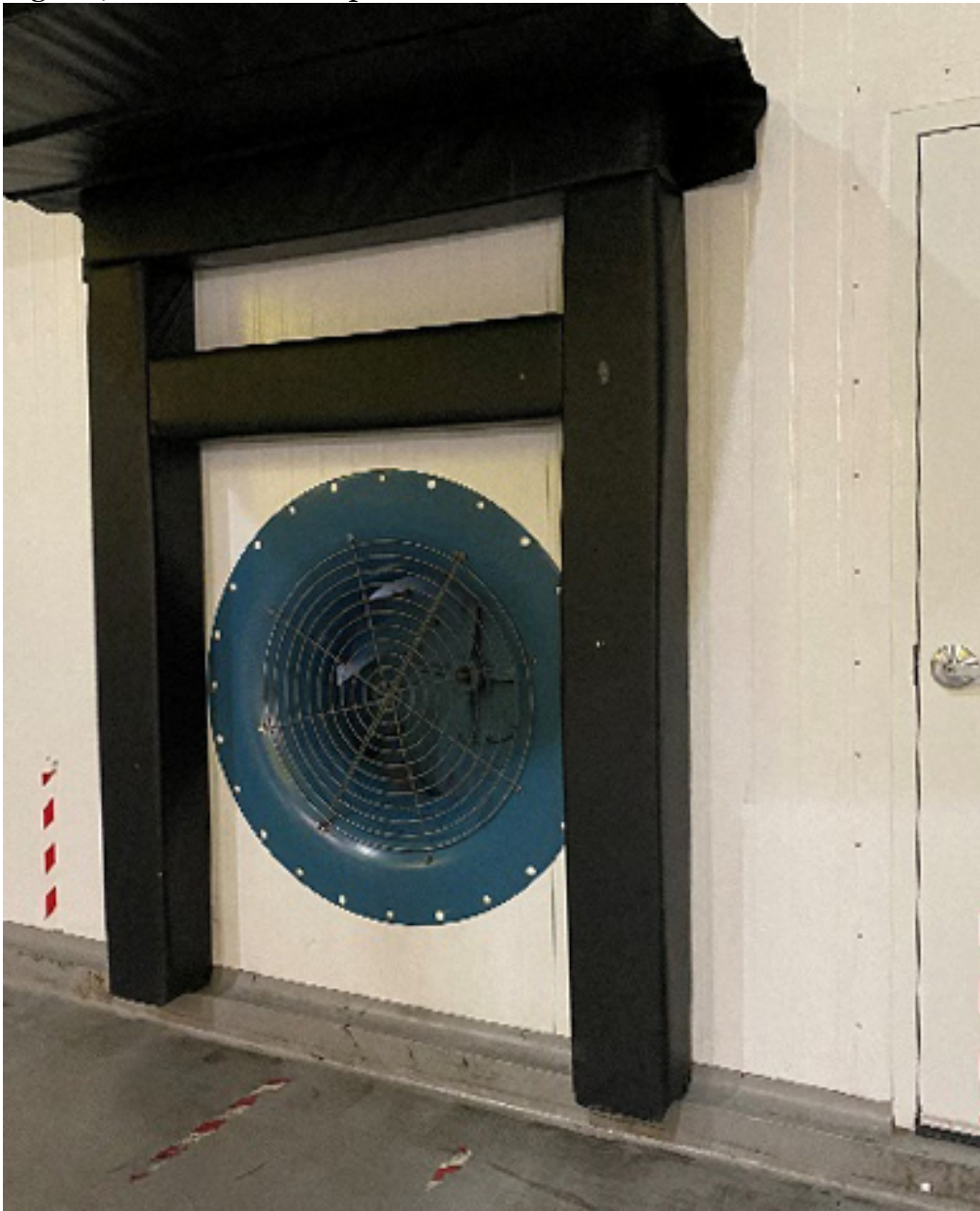
Figure 7. Forced-Air Setup Within a Cold Room.
