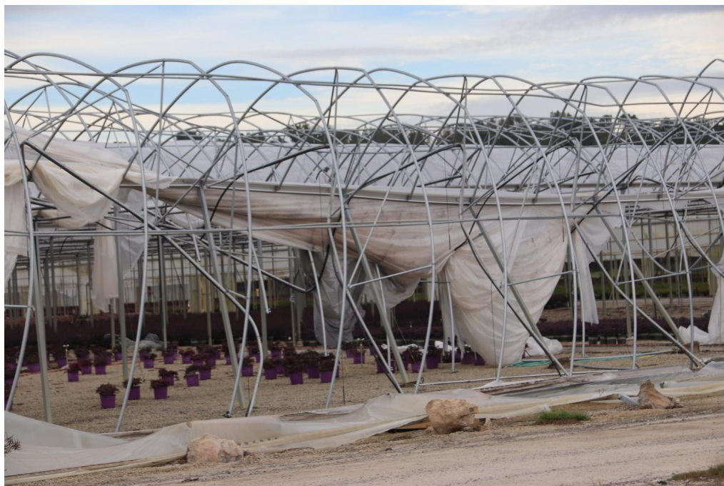
Figure 5. Greenhouse Roof Damaged by High Winds (at McCorkle Nursery). Photo: Georgia Farm Bureau.
