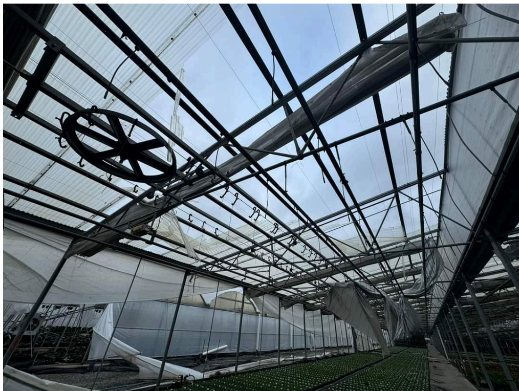
Figure 2. Roof and Structural Damage. Photo: Sunbelt Greenhouse.
