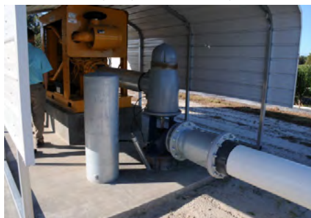
Figure 3. The wellhead should be inspected prior to a freezing event.
