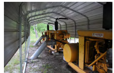
Figure 5. Diesel-powered prime movers for irrigation pumps.
