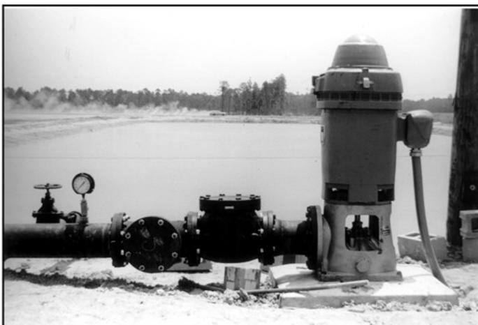
**Figure 14.** Large agricultural well with electric motor.
