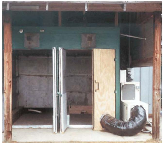
**Figure 4. Conventional barn (left) beside the heat-pump barn (right) with coupled heat-pump-dehumidifier**
