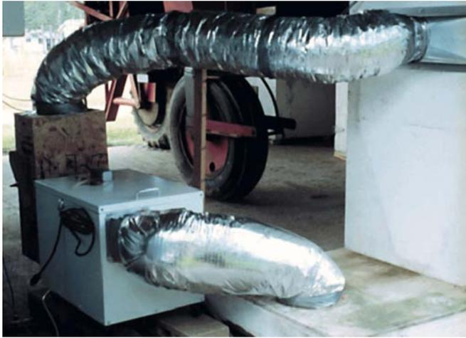
**Figure 3. Heat-pump-dehumidifier coupled to the two-rack barn via flexible ducts.**
